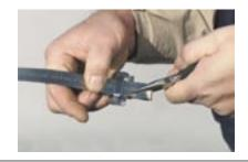
■ 2. Band attaching base to pipeline.
